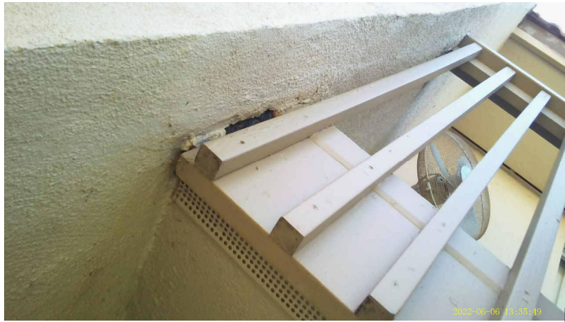
4086#6: Exposed wall framing building wrap
