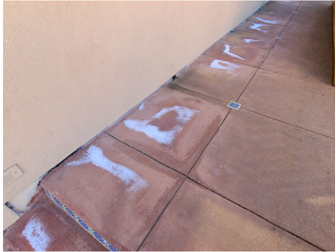
4050 Concrete Efflorescence
