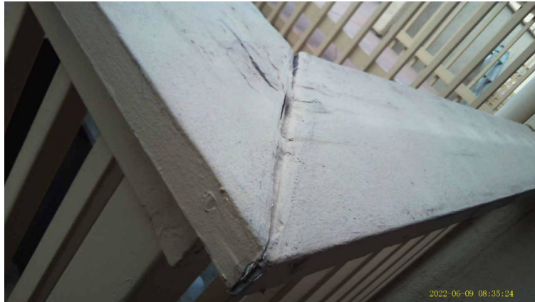
4050 #1: Handrail Dryrot
